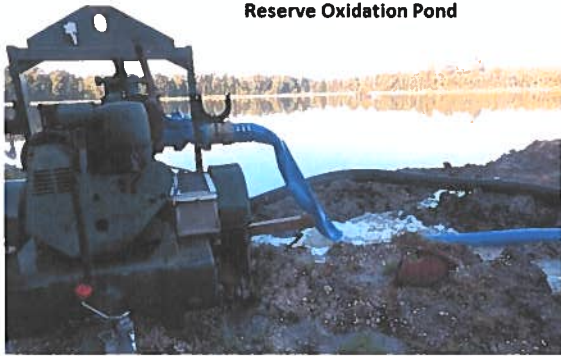
Reserve Oxidation Pond
