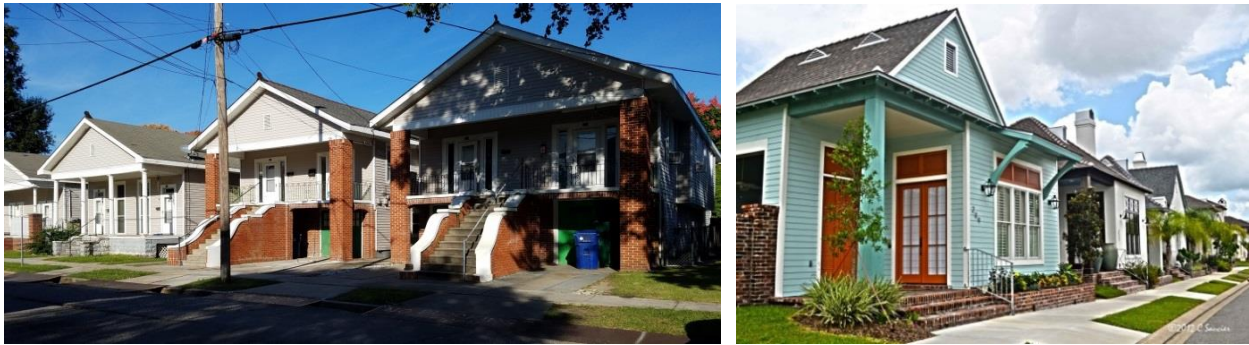
Figure 8-2: Single Family Residential - Algiers, LA (left); River Ranch, LA (right)
