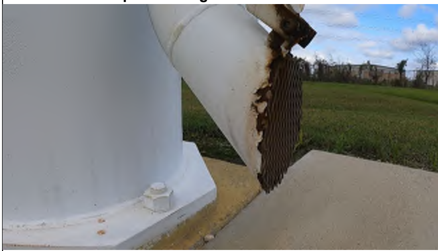
# 68: Overflow Pipe Discharge
