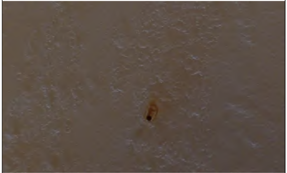
# 14: Interior – Shell Corrosion
