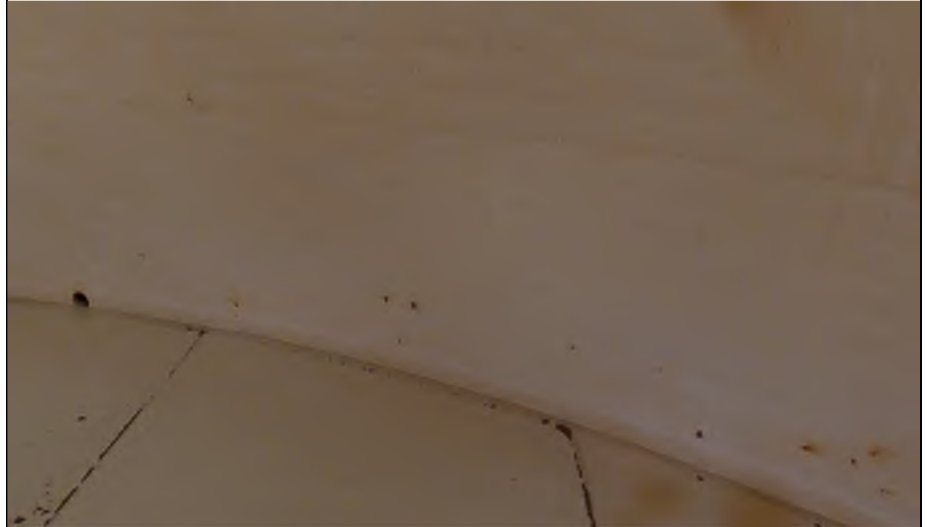
# 15: Interior – Shell Corrosion Areas
