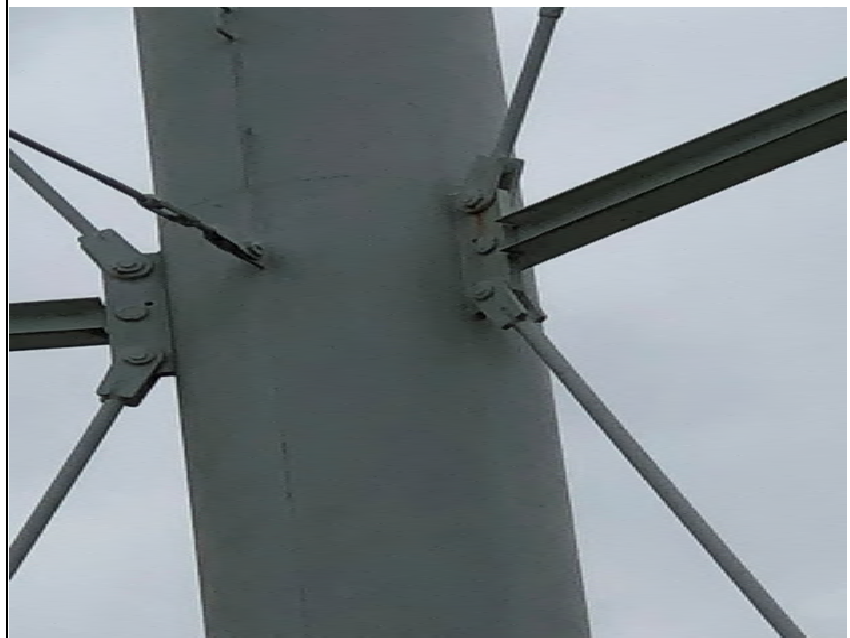
# 57: Lower Strut &amp; Brace Rod Connections
