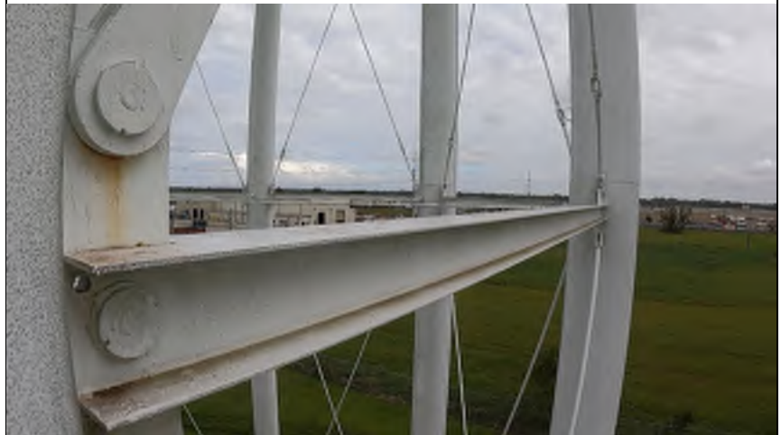
# 57: Lower Strut &amp; Brace Rod Connections
