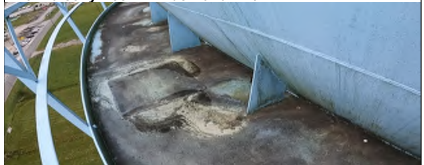
# 47: Balcony Deck - Pitting and Water Ponding
