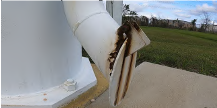
# 68: Overflow Pipe Discharge
