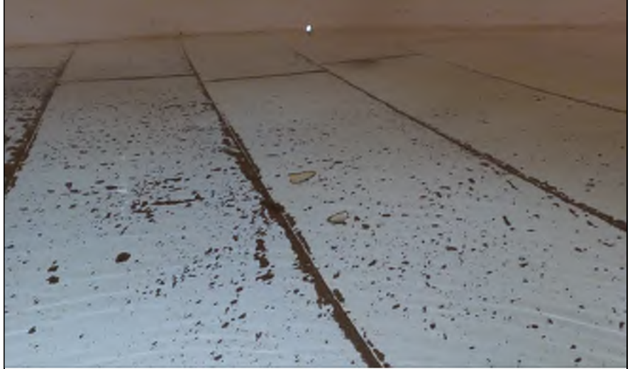
# 26: Interior – Floor Corrosion
