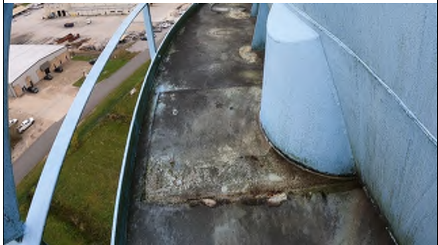
# 45: Balcony Deck - Pitting & Corrosion
