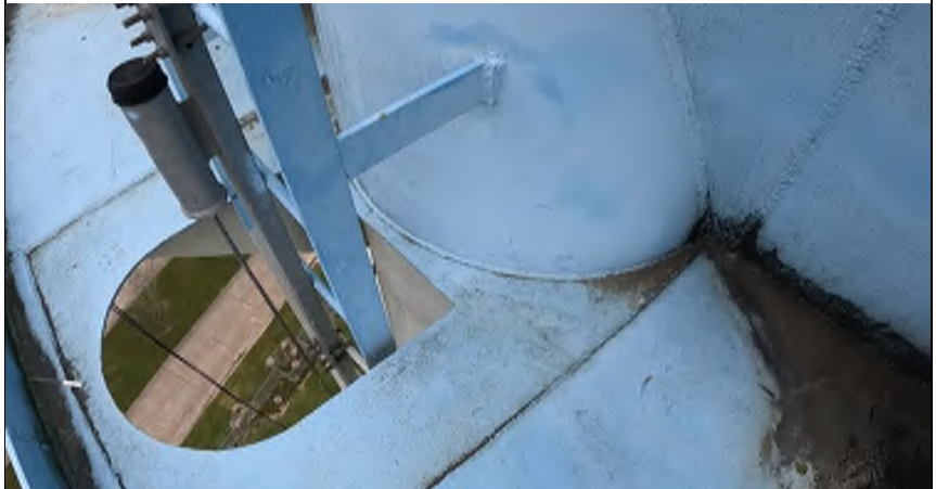
# 50: Balcony Handrail Attachment
