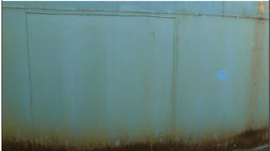
# 42: Exterior – Shell Top Coat Loss
