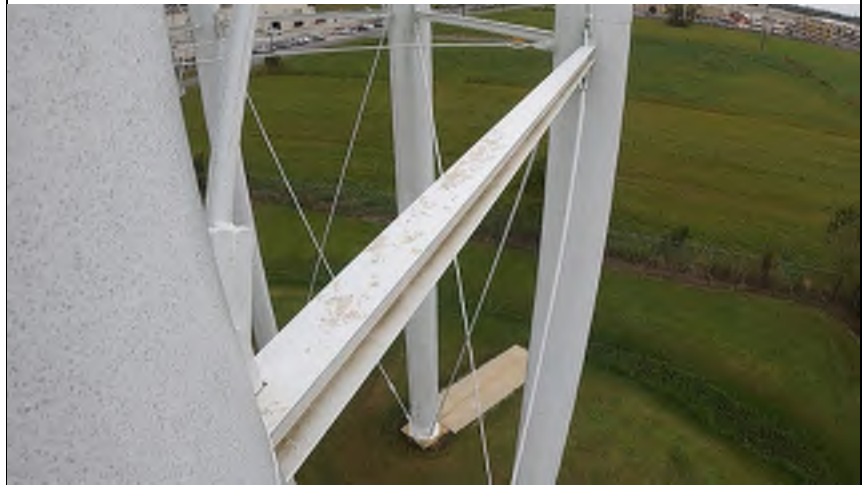
# 56: Lower Strut to Leg Connection
