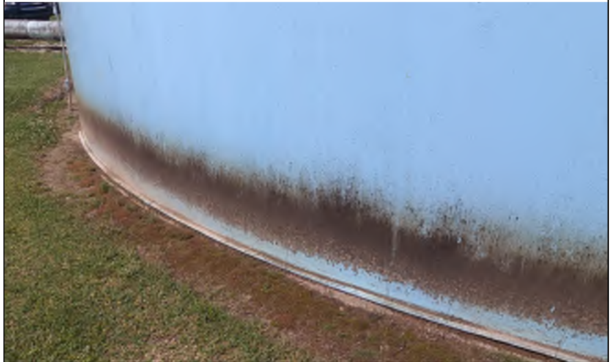
# 39: Exterior - Shell Top Coat Loss
