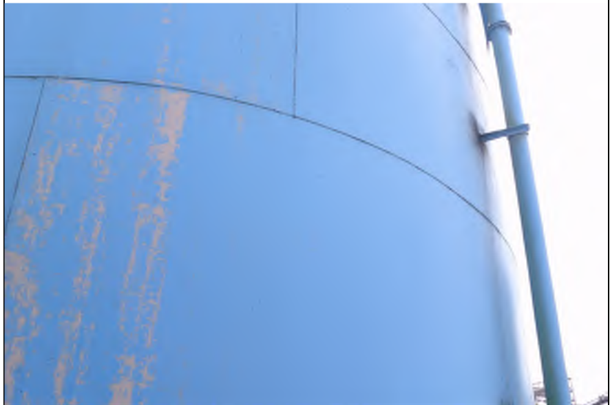
# 42: Exterior – Shell Top Coat Loss
