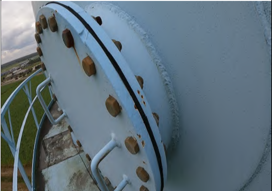
# 40: Exterior Shell Manhole
