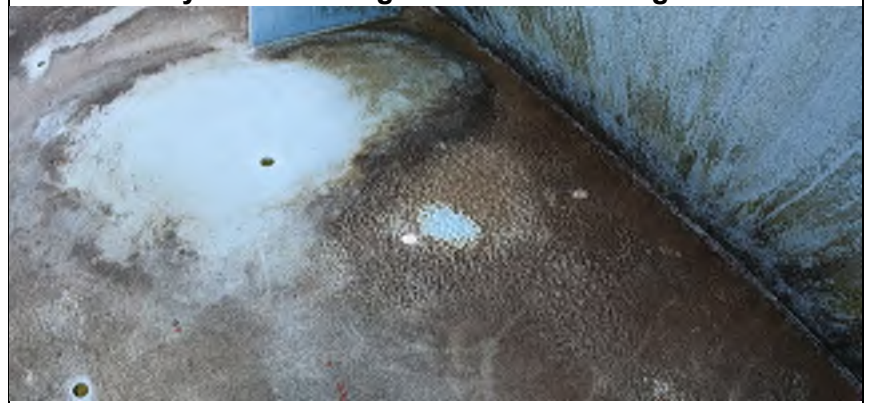
# 48: Balcony Deck, Pitting and Water Ponding
