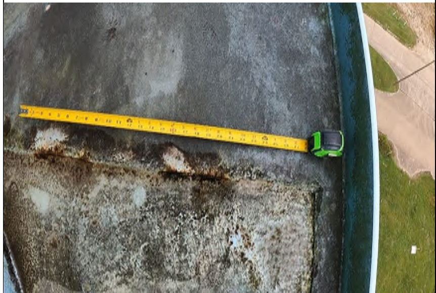
# 45: Balcony Deck - Pitting & Corrosion
