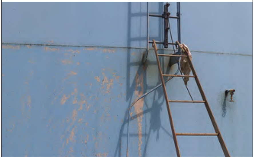
# 39: Exterior - Shell Top Coat Loss
