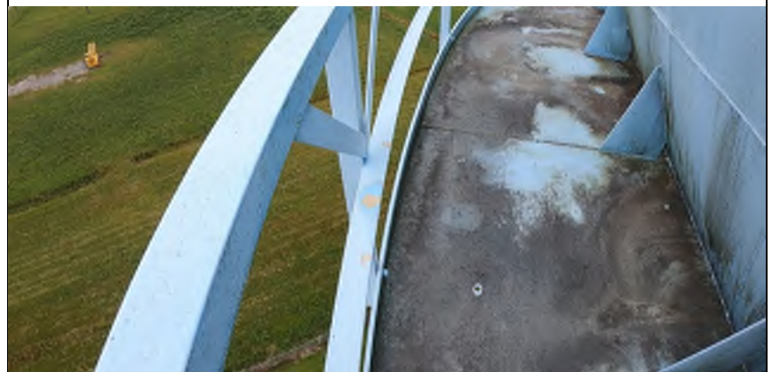
# 48: Balcony Deck, Pitting and Water Ponding
