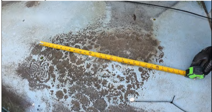
# 44: Balcony Deck - Pitting & Corrosion
