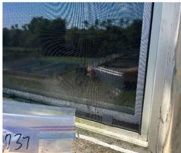
Samples 037 / 038 Window Caulk Site/Office Building, 2 nd Floor Exterior @ North No asbestos detected
