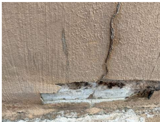
Samples 058 / 059 Stucco Treatment Units No asbestos detected
