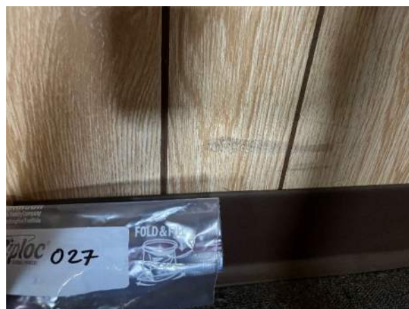
Samples 027 / 028 Dark Brown Baseboard & Mastic Site/Office Building, 2 nd Floor No asbestos detected
