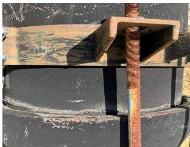
Samples 056 / 057 Black Pipe Coating Exterior No asbestos detected
