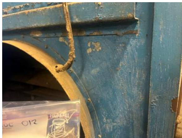
Samples # 012 / 013 White Fabric Gasket Site/Office Building, 1 st Floor @ Blower 4 No asbestos detected
