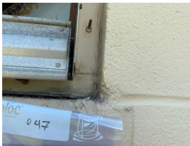
Samples 046 / 047 Colorless Misc. Caulk Site/Office Building, Exterior No asbestos detected
