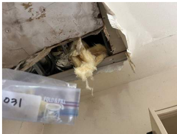
Samples 031 / 032 Fiberglass Insulation Site/Office Building, 2 nd Floor No asbestos detected
