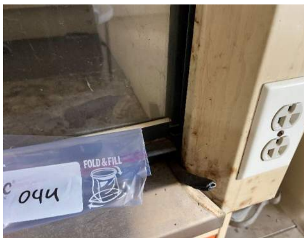
Samples 044 / 045 Black Rubber Seal Site/Office Building, 2 nd Floor @ Lab Hood No asbestos detected
