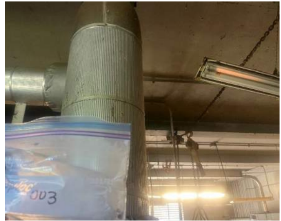
Samples # 003 / 004 / 005 Chalky Insulation w/ Silver Metal Jacket Site/Office Building, 1 st Floor @ Generator No asbestos detected
