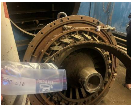
Samples # 010 / 011 Black Foam Gasket Site/Office Building, 1 st Floor @ Blower 4 No asbestos detected
