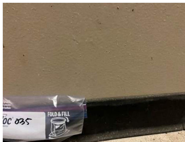
Samples 035 / 036 Black Baseboard & Mastic Site/Office Building, 2 nd Floor @ Stairs No asbestos detected
