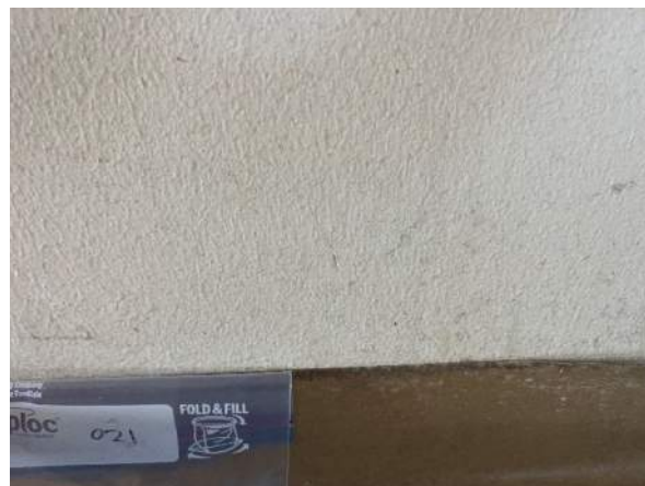
Samples 021 / 022 Tan Baseboard & Mastic Site/Office Building, 2 nd Floor Lab No asbestos detected
