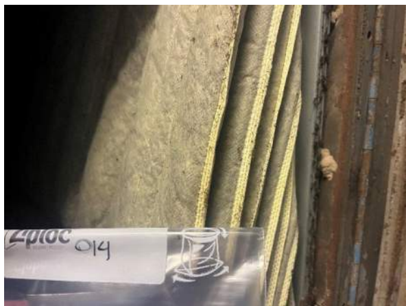
Samples 014 / 015 Gray Air Filter Insulation Site/Office Building, 1 st Floor @ Blower 3 No asbestos detected
