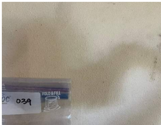
Samples 039 / 040 / 041 Sheetrock & Texture Site/Office Building, 2 nd Floor No asbestos detected
