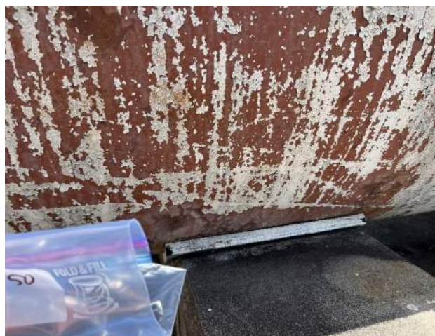
Samples 050 / 051 Rubber Tank Pad Site/Office Building, Exterior @ Tanks No asbestos detected
