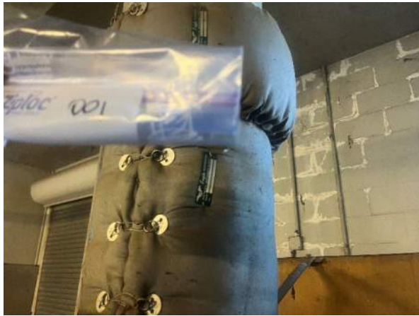
Samples # 001 / 002 Gray Fabric Jacket Insulation Site/Office Building, 1 st Floor @ Generator No asbestos detected
